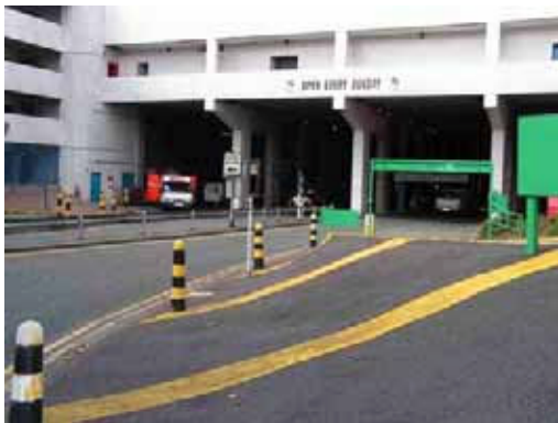
Photo 5: Service roads underneath mall
