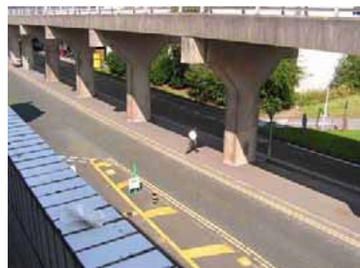
Photo 3: Pedestrian crossing road at ground level
