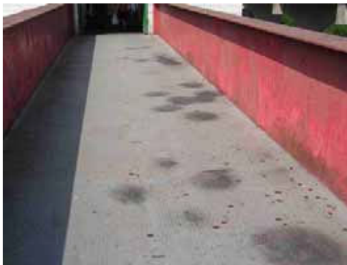
Photo 20: Surface of footbridge from East Lane House.
