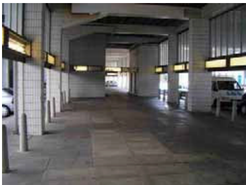
Photo 15: Disused former Regional bus station
