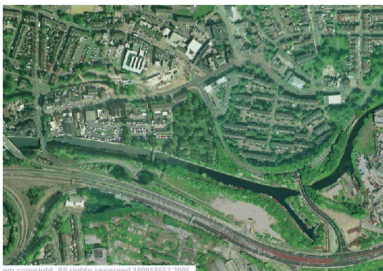
Aerial view of Town Centre in 2000 showing new access road from Daresbury expressway (bottom right) and construction of new bus station (top centre left).
