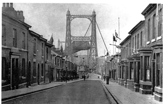
View of the approach to the Transporter Bridge, which provided the sole vehicular link between Runcorn and Widnes until 1961.
