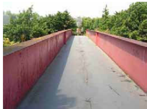
Photo 2: Footbridge towards Asda
